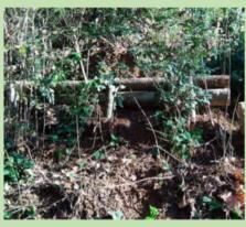
**4) Brush layer:** a series of steps excavated on the slope in which bundles of plant cuttings are inserted to promote slope protection and revegetation.
