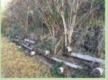
2) Live Grating: a lattice made of timber logs and anchored at the base and to the slope, acting as skin on the slope.
